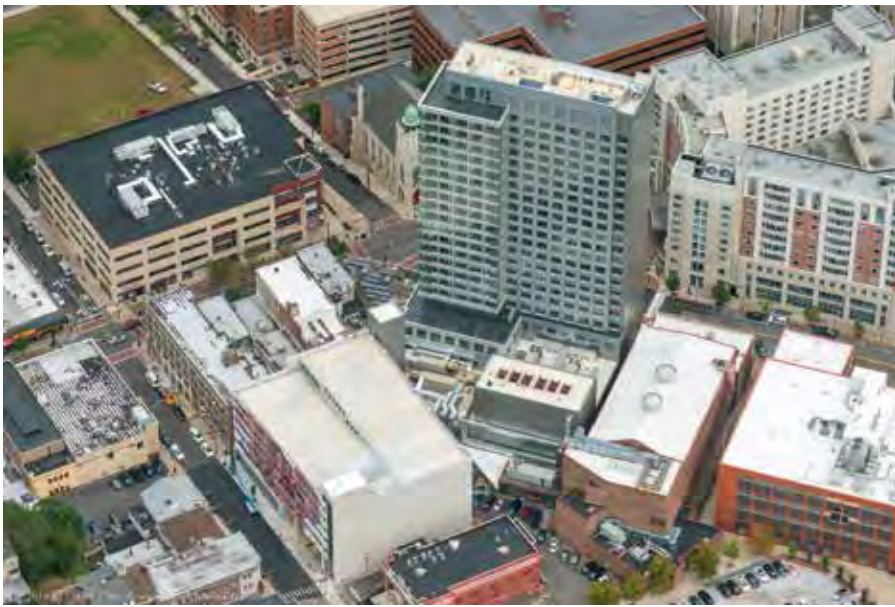
The New Brunswick Performing Arts Center, a 23-story building that includes apartments and two theatres, opened in September 2019 in New Jersey. | Courtesy of Elkus Manfredi Architects.
