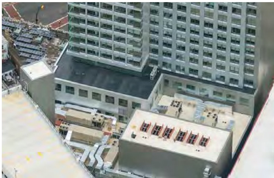
The project includes acoustical roof hatches manufactured by The BILCO Company, which limit noise intrusion while also allowing for the release of smoke, heat, and gases in a burning building. | Courtesy of Elkus Manfredi Architects.
